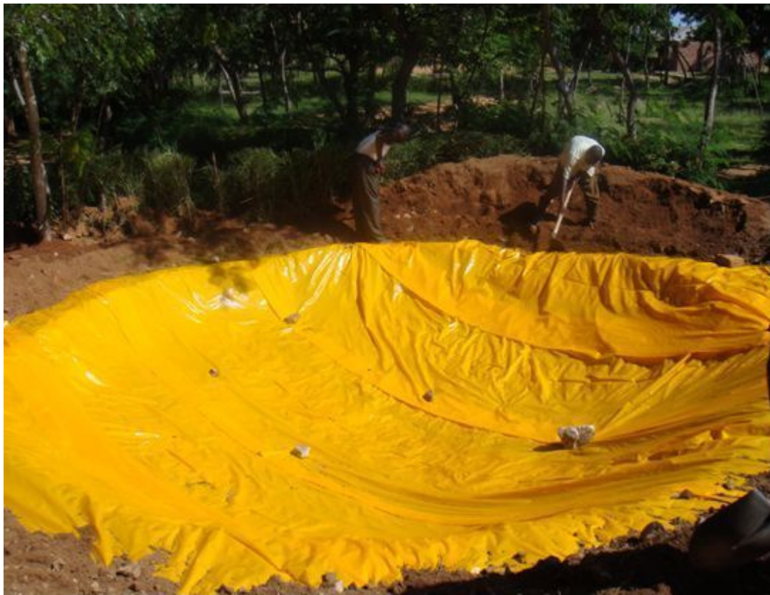
Figure 4. Completed water pan (A) at Nyangere Secondary School lined with yellow polyethylene material.
